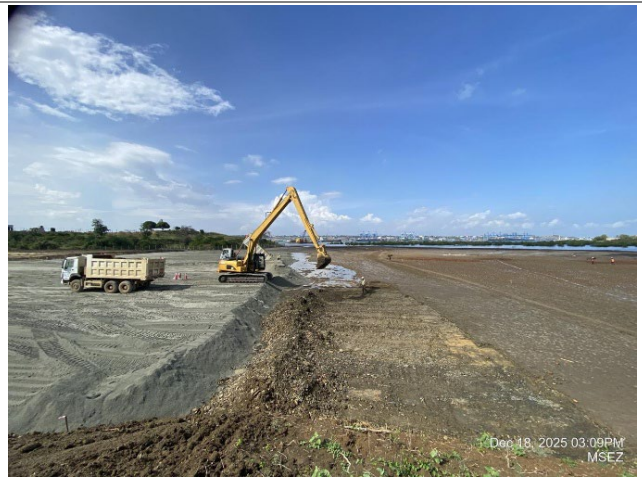
Topsoil stripping at Reclamation Yard
