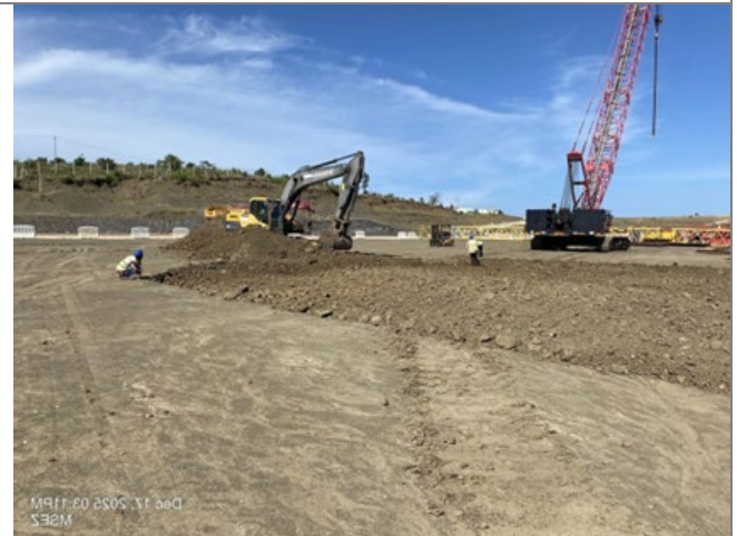
Precast yard preparation
