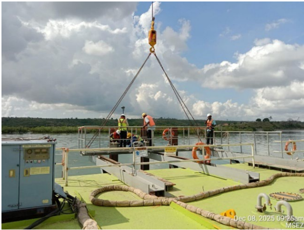
Setting out of Survey Platform 2
