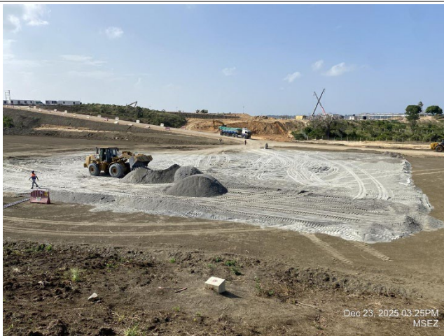
Rock sand stock piling
