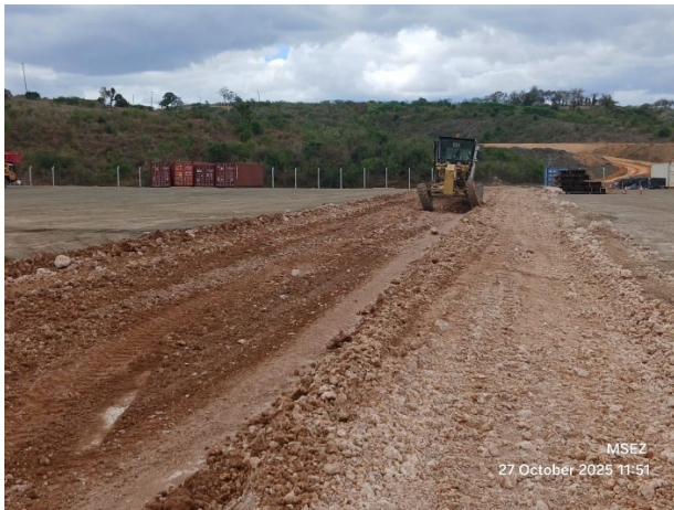
Temporary Access Road Construction
