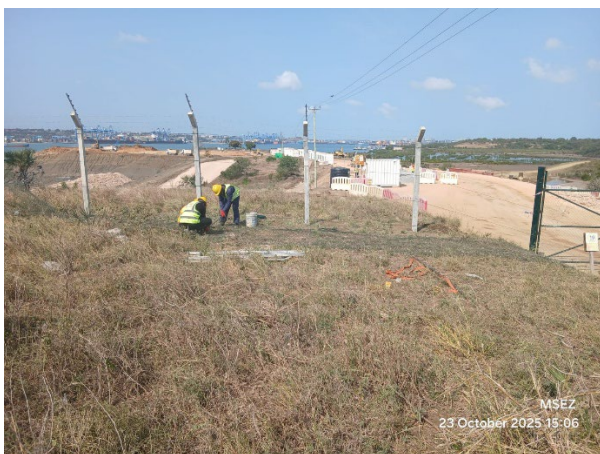
Temporary Access Road Construction
