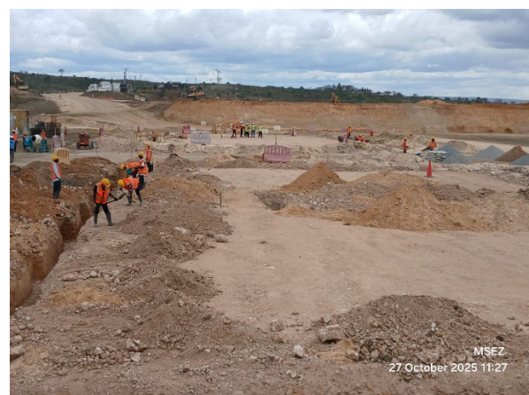
Contractor's Office & Canteen Construction
