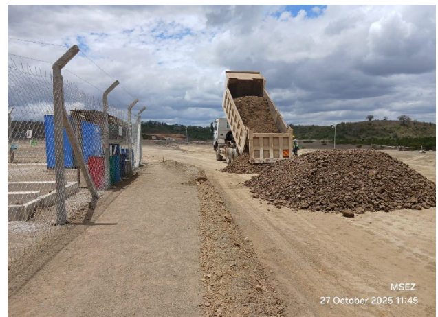
Temporary Access Road Construction
