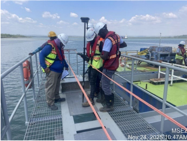
Survey Platform 1 Construction
