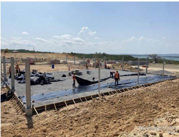
Contractor Office: Laying of DPM & Formwork Installation
