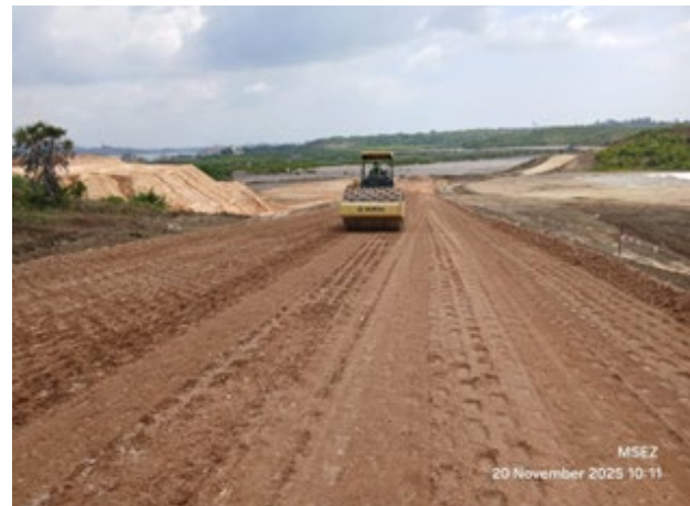
Temporary Access Road: Compacting 1 st Later Wearing Course ACS-05
