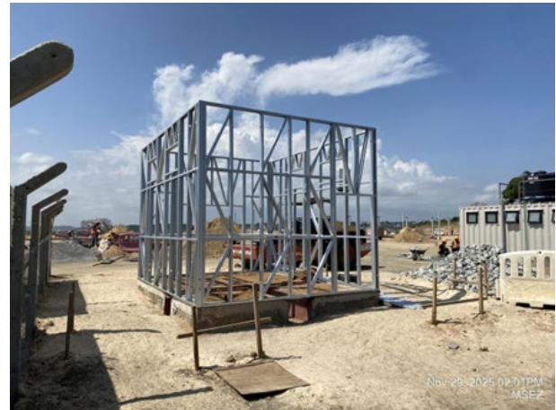
Powerhouse LGS Panel Assembly
