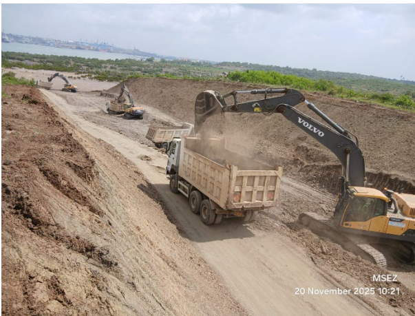
Temporary Access Road: Cutting and Hauling Material ACS-10
