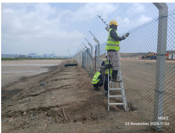
Perimeter Fencing: Installation of Chain Link Fencing Between Point 1 and 30
