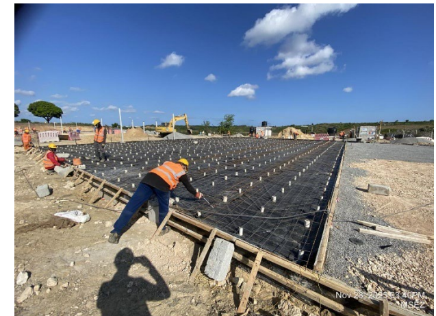
Canteen: DPM and BRC Installation
