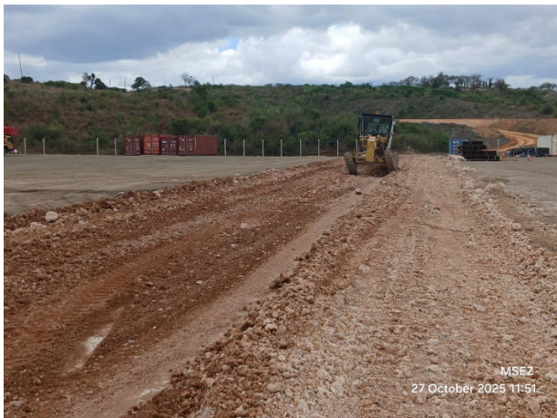
Temporary Access Road Construction
