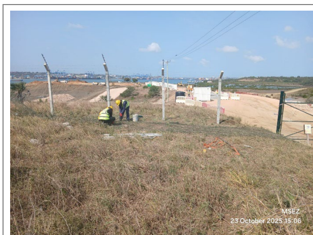
Temporary Access Road Construction
