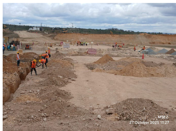
Contractor's Office & Canteen Construction
