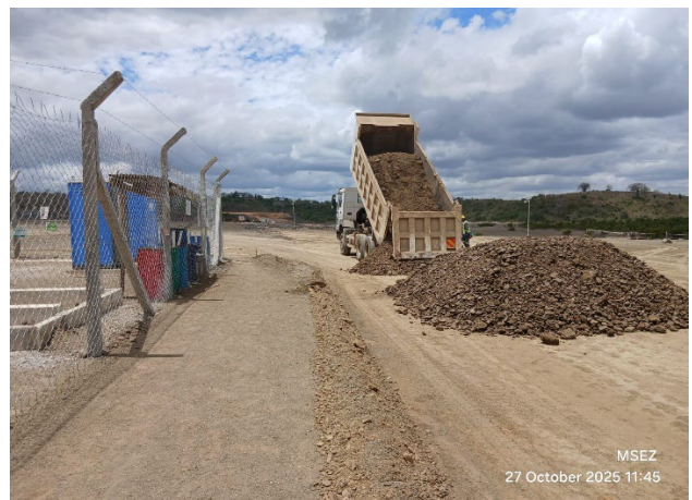
Temporary Access Road Construction
