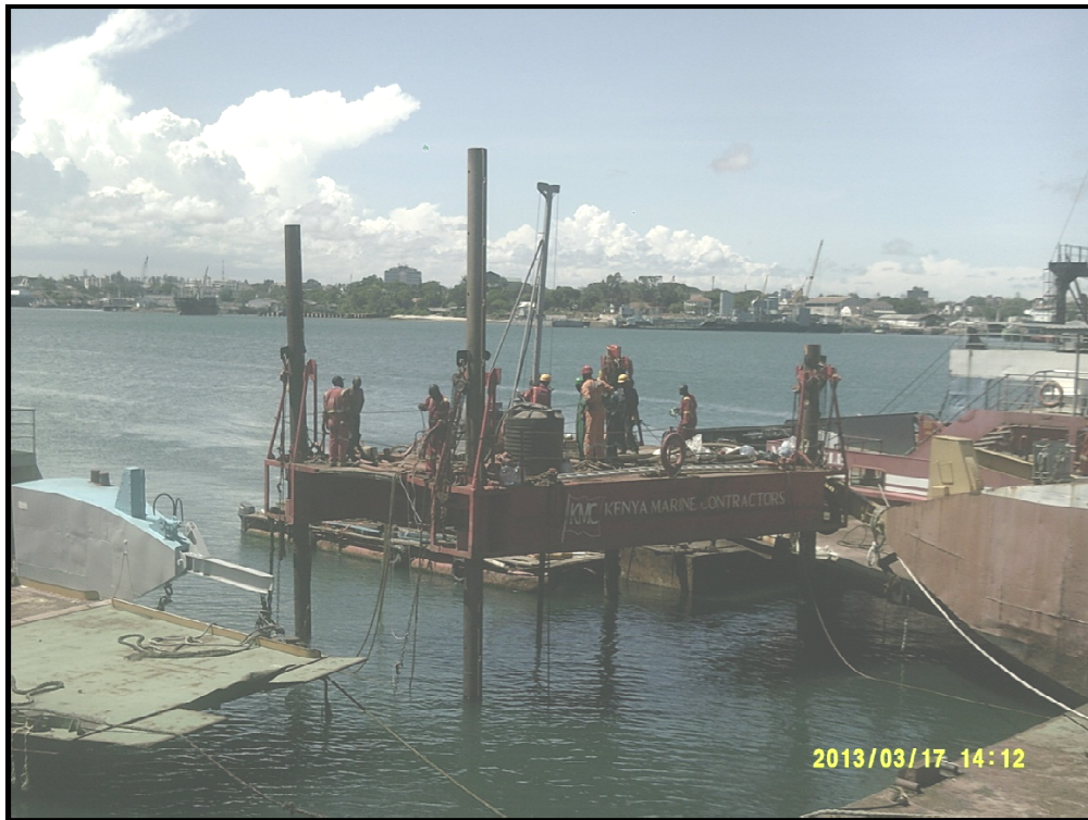
GEOTECHNICAL DRILLING AT BH 3 LOCATION
