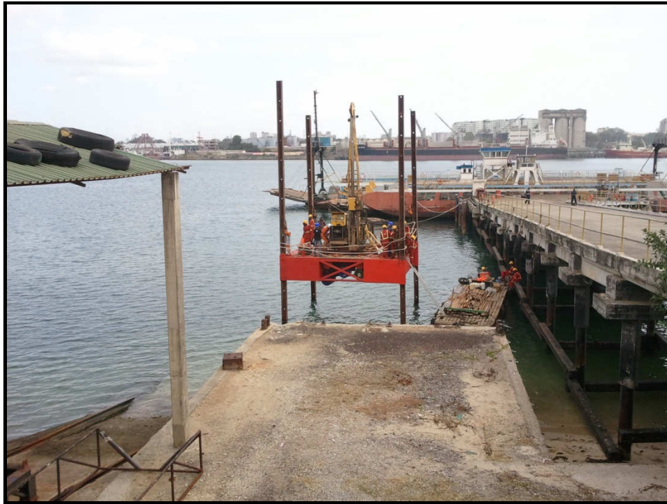
GEOTECHNICAL DRILLING AT BH 1 LOCATION
